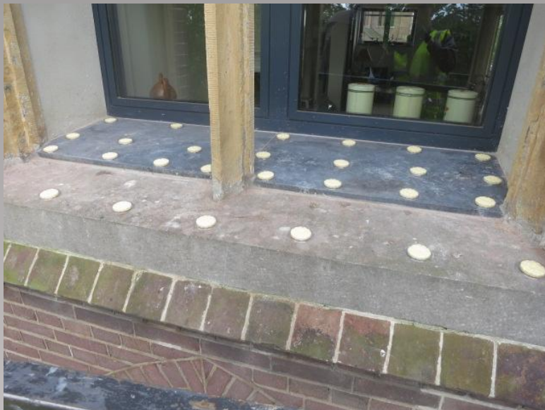
On the east side of the chapel, six window ledges were cleaned and treated with Bird Free as shown above.
