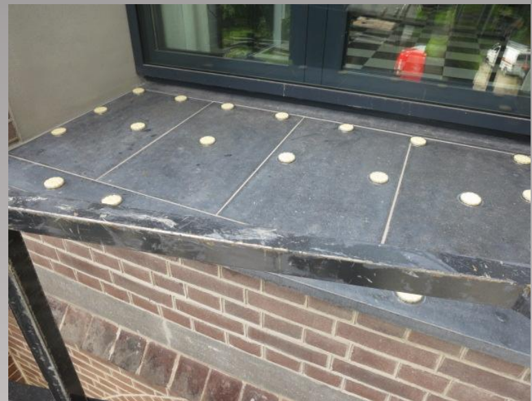
On the east side of the chapel, six window ledges were cleaned and treated with Bird Free as shown above.
